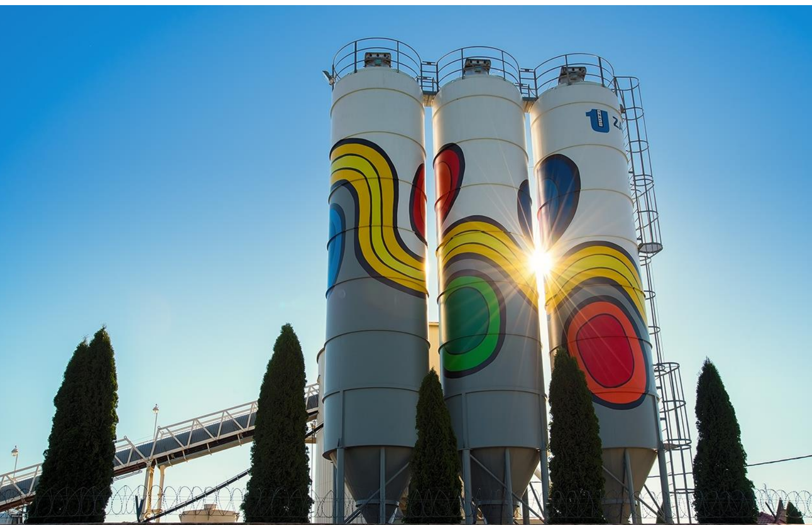
Ready mix-batch plant, Hlohovec, Slovakia
